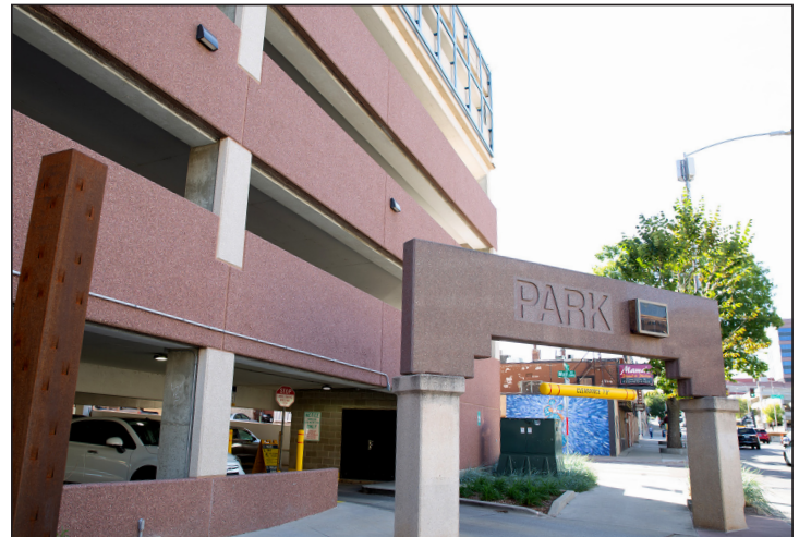
11th Street Parking Ramp Next to SAM Transit Bus Depot
