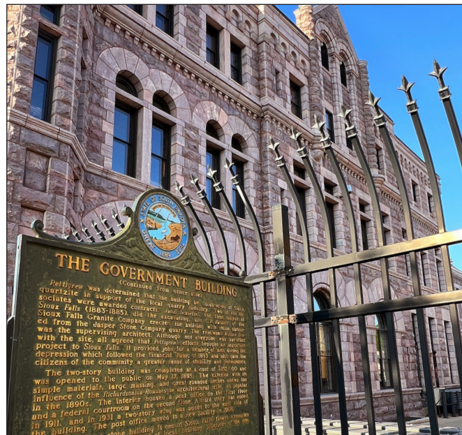
Federal Building and United States Courthouse
