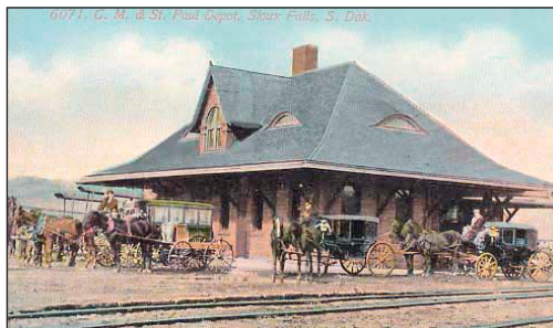
Depot on 5th Street and Phillips Avenue, 1900s
